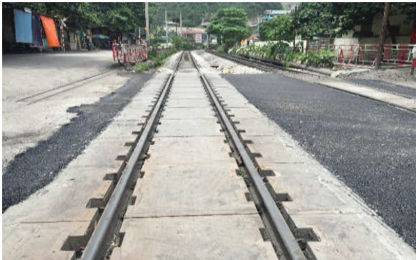
Prestressed concrete slab installed at the entrance to Mong Duong coal mine - Cam Pha - Quang Ninh.
