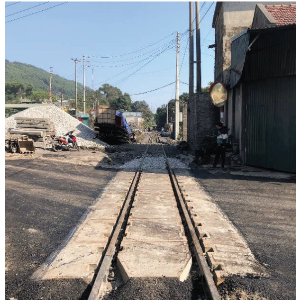
Prestressed concrete slab installed at the entrance to Deo Nai coal mine - Cam Pha - Quang Ninh
