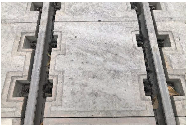
Prestressed concrete slab installed at the entrance to Coc 6 coal mine - Cam Pha - Quang Ninh.
